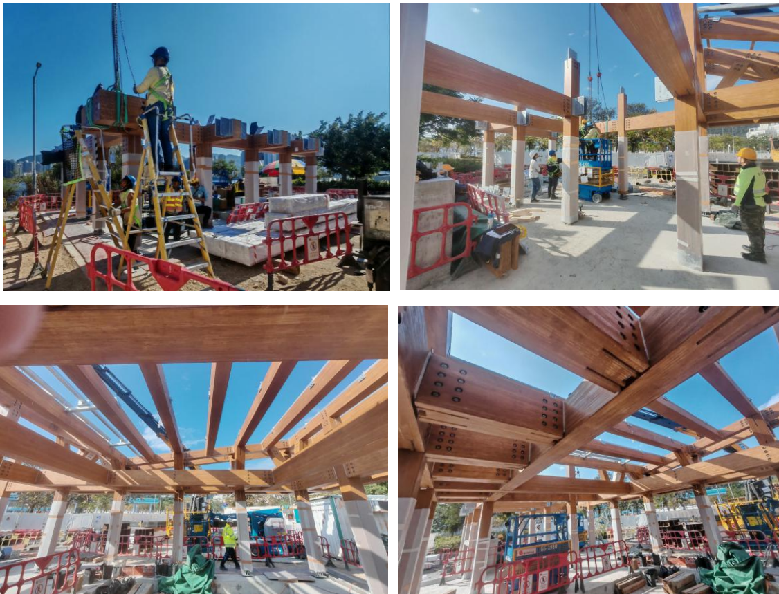
Fig. 14. Assembly of prefabricated components
