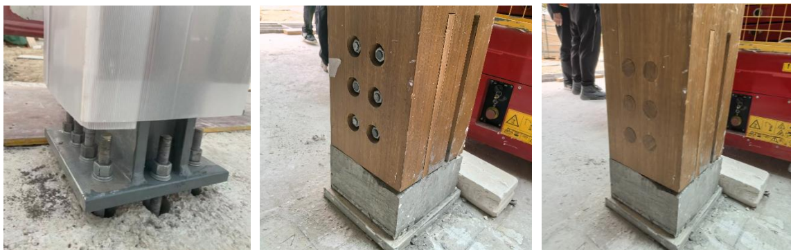
Fig. 12. Connections for the bottom of columns
