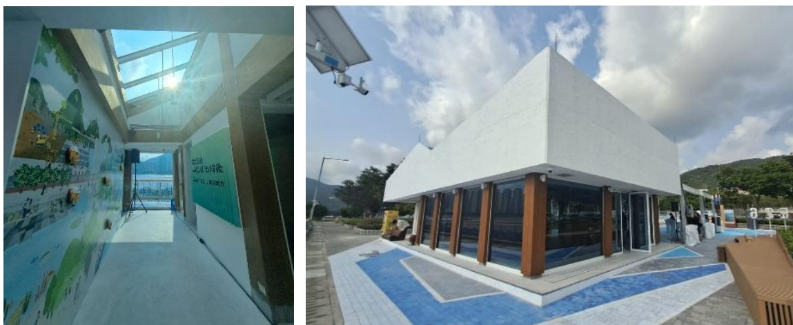
Fig. 17. The completed building
