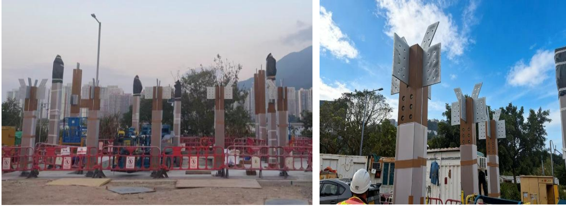
Fig. 13. Construction of columns
