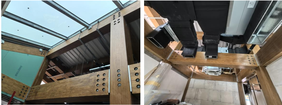
Fig. 16. Bolted connections
