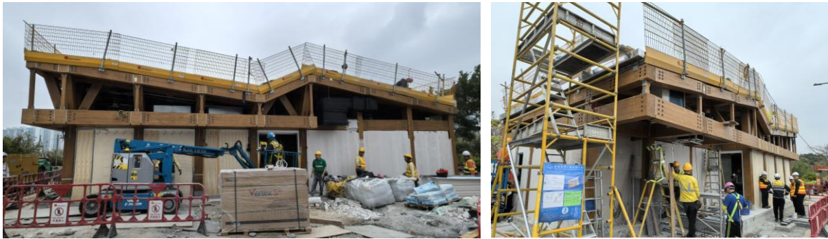
Fig. 15. Main structure frame
